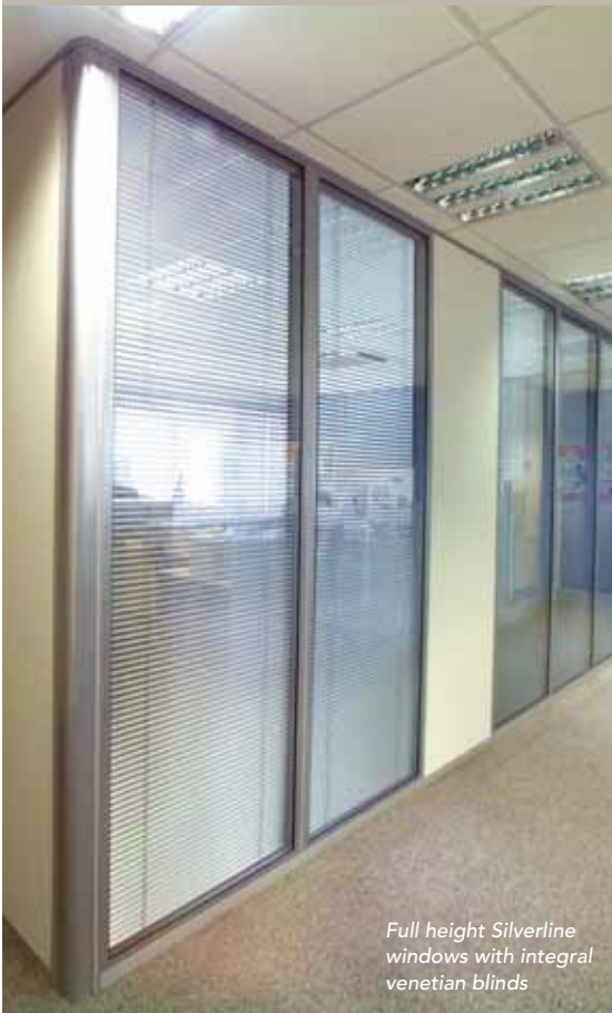
Door head height pre-assembled windows with integrated venetian blinds and veneered doors
